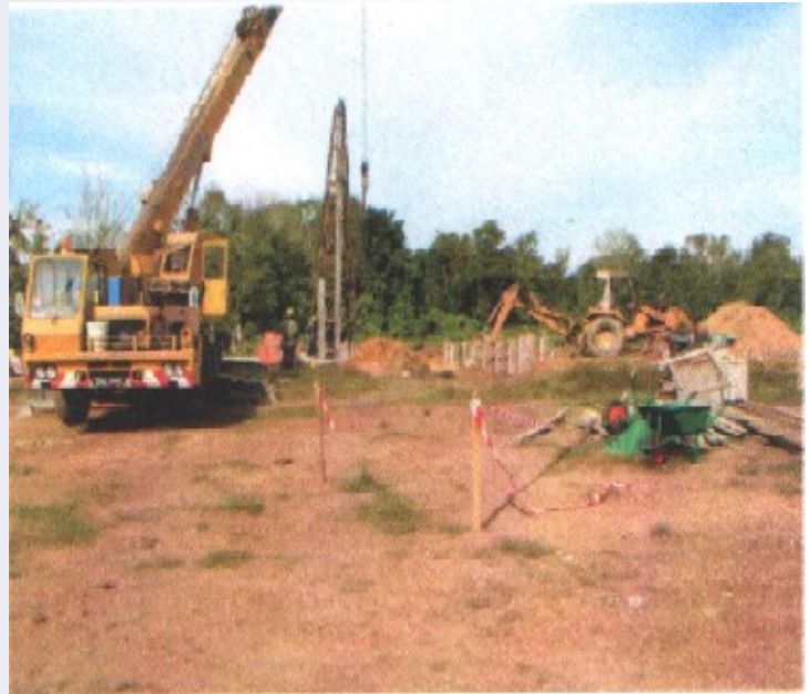
PILING FOR BTS TOWER (LITO)
