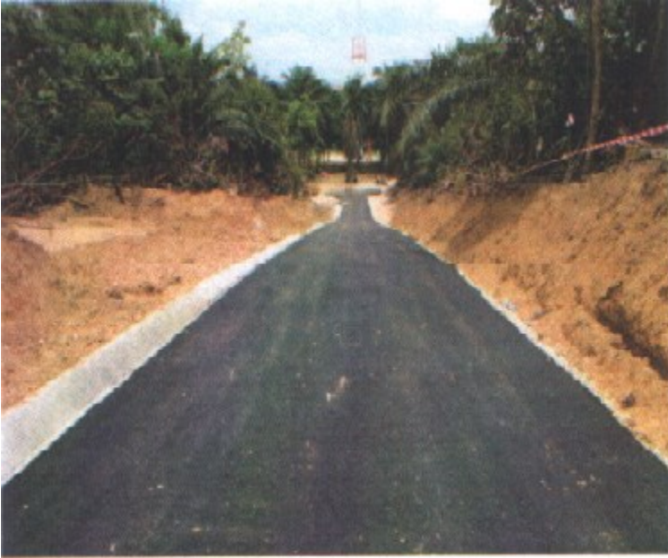
PREMIX ROAD CONSTRUCTION (ANTQ)
