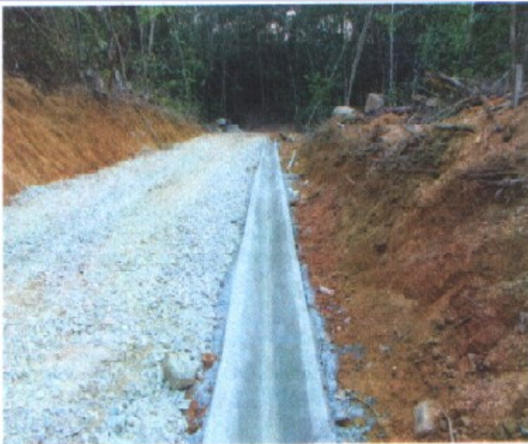
CONCRETE DRAIN CONSTRUCTION (ANTQ)
