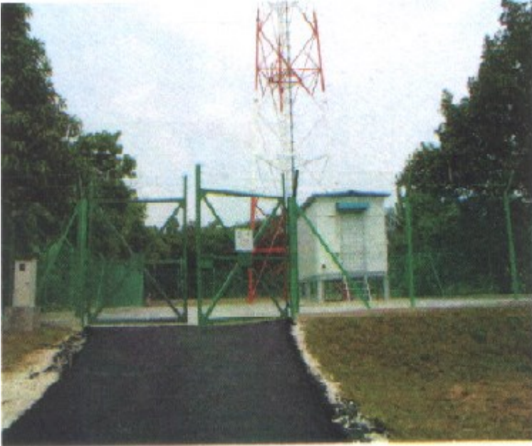
FENCING, GATE, TURFING & TNB PLINTH (MBAI)
