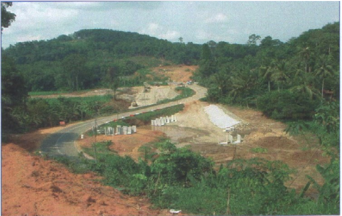
ROCK TOE AND BOX CULVERTS
