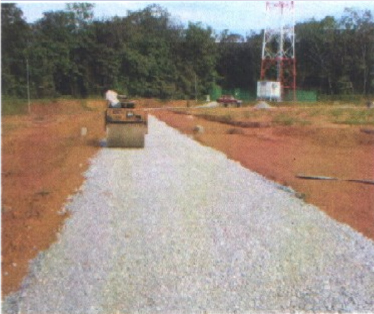
CRUSHER RUN ROAD CONSTRUCTION (IMAH)
