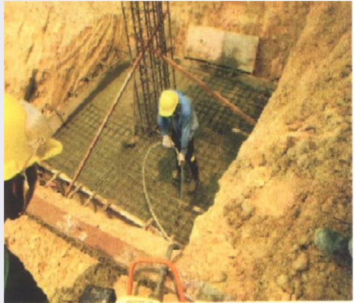
BTS TOWER FOOTING CONSTRUCTION (SPAT)
