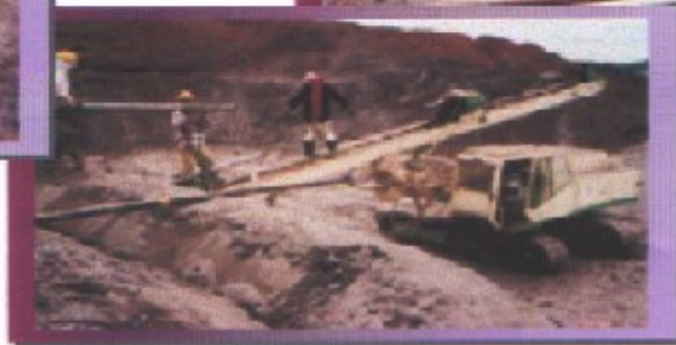
EARTHWORK AT PRECINCT 2, PUTRAJAYA.
