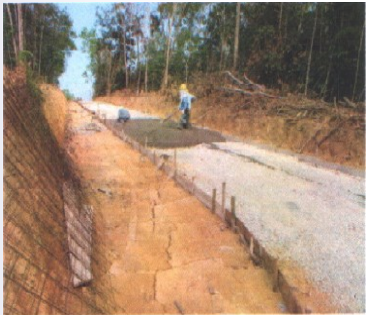
CONCRETE ROAD CONSTRUCTION (ANTQ)
